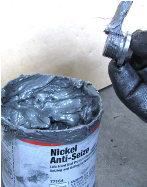
Fig. D-1. Apply nickel-based anti-seize lubricant to the screw threads of valve seat.
